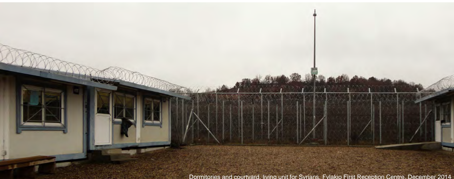
Dormitories and courtyard, living unit for Syrians, Fylakio First Reception Centre, December 2014
